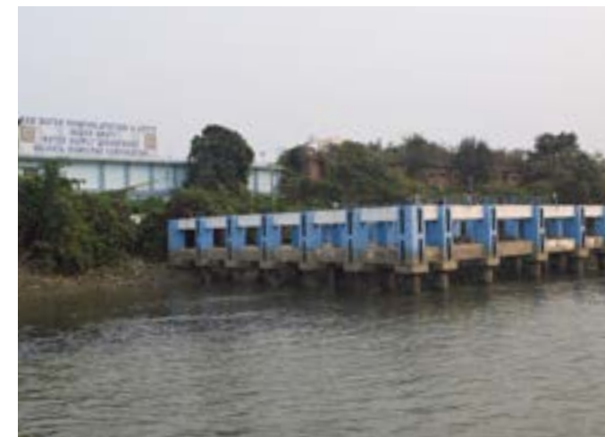
Above Image: Raw water pipping station at Mayer Ghat
